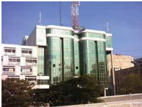
Mobile phone company Telenor in Pakistan is protected by Kentec's extinguishant control and release system
